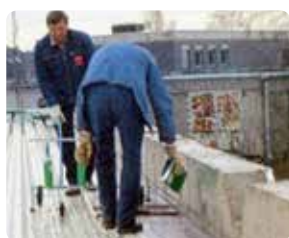
Adhesive consumption in edge and corner areas regularly approx. 120 g/m 2 approx. 100 g/m 2
