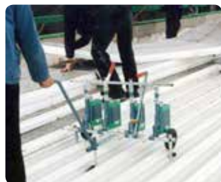
Adhesion of rigid polystyrene foam on plastic-coated trapezoidal sheets.
