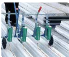
Adhesive consumption on flat surfaces regularly approx. 100 g/m 2
